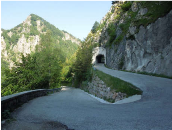
Road of the Campogrosso pass, south slope
